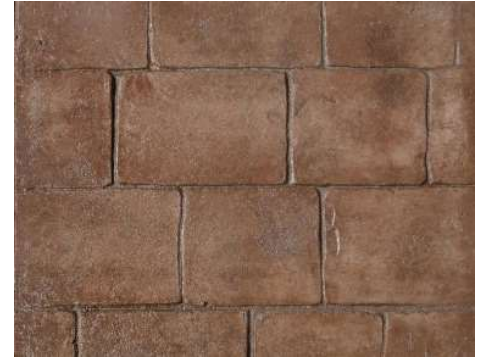
foundation stamped concrete
